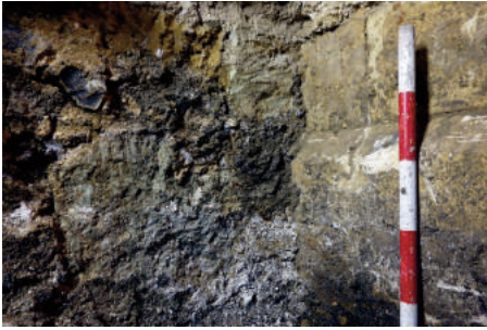
Elevation view looking south east, showing (left) the Greensand footings of the 1398 rear wall of the ambulatory abutting (right) the exterior face of the north wall of the north transept
