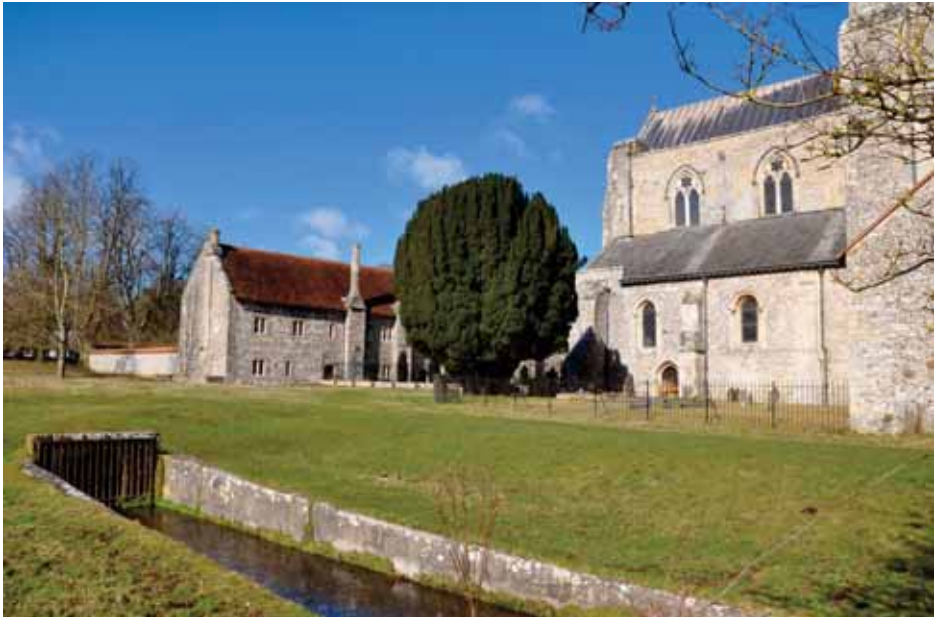
The eighteenth-century bricked conduit that brings the Lockburn from behind the Brothers' quarters into the Park
